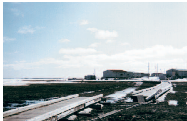
Fig. 15.14. Boardwalk damaged by storm surge flooding, Kipnuk, Alaska (photo by Mike Marcaurele).
