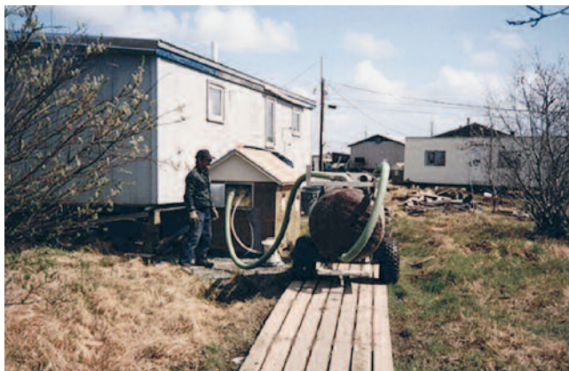
Fig. 15.16. Small sewage haul system, Mekoryuk, Alaska (photo by Mark Baron).
