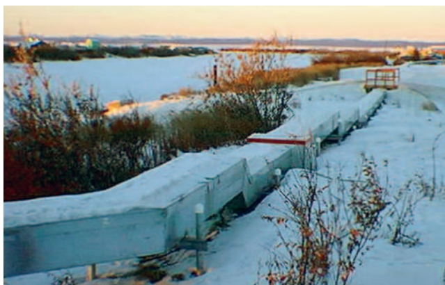
Fig. 15.13. Aboveground water and sewer utilidor, Selawik, Alaska (photo by John Warren).
