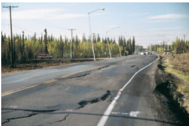
Fig. 16.20. Typical embankment cracking and differential thaw settlement in the discontinuous permafrost zone of Interior Alaska (Photo: Larry Hinzman, University of Alaska, Fairbanks).
