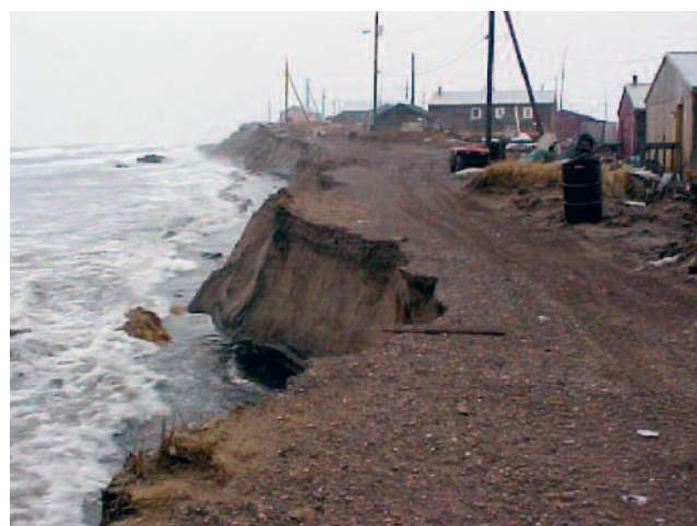
Fig. 15.18. Access road damage by coastal erosion, Shishmaref, Alaska (photo by Tony Weyionanna).
